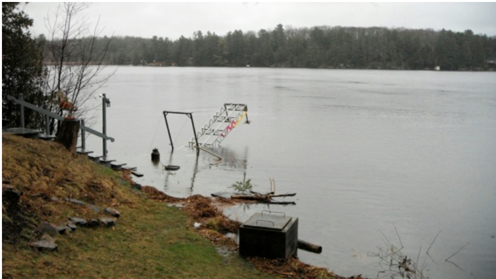
Moore Lake: Overbank flooding of shoreline infrastructure
