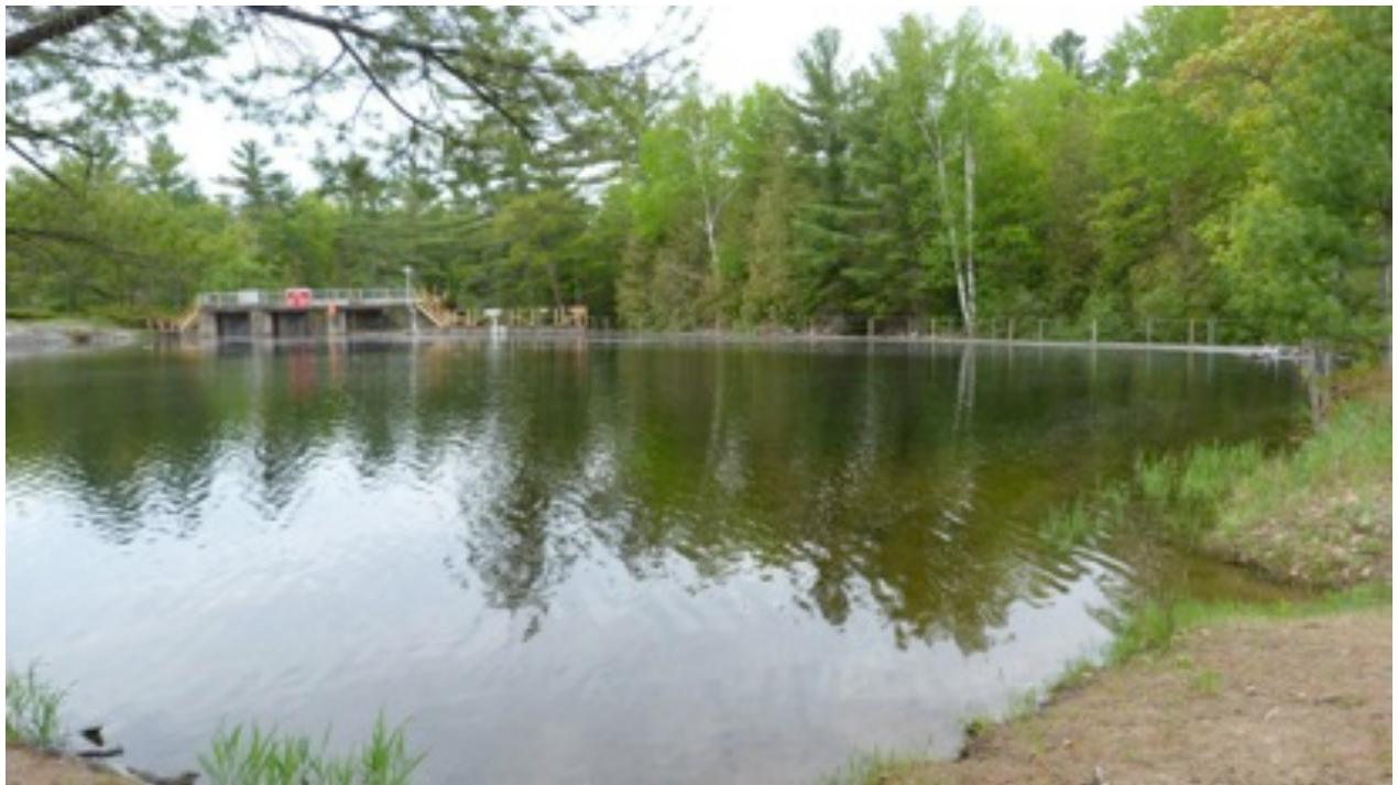
Mississagua dam at capacity
