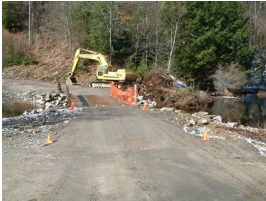
Repairing the Invader Lane Causeway (Redstone Lake) with a temporary bridge
