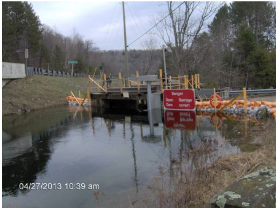
Buttermilk Falls dam sandbagged to prevent overflow
